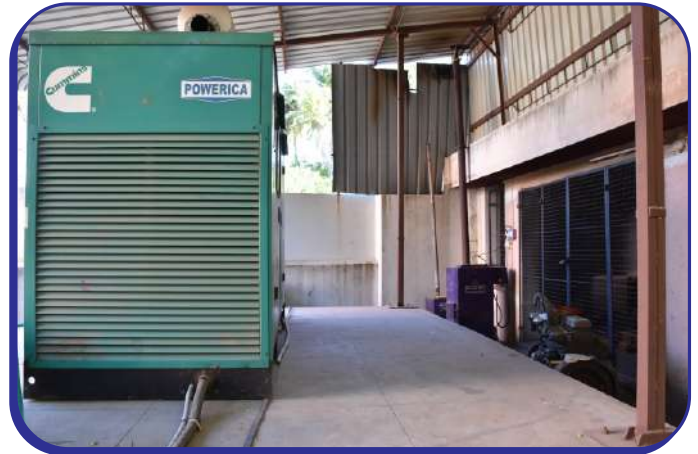
Generator for Hostel
