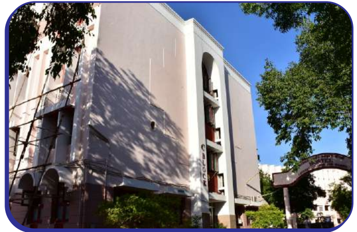
Administrative Block - C Block
