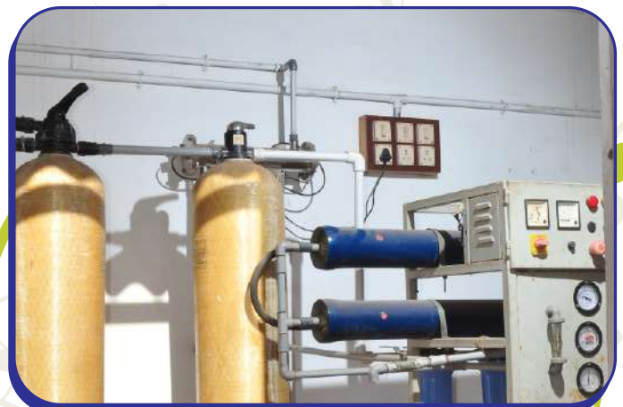
RO Water System
